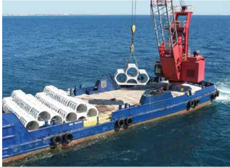
The project was 100% grant-funded from the Natural Resource Damage Assessment
